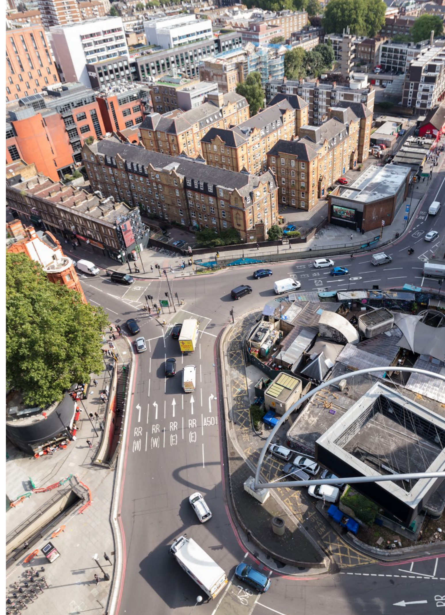
The superstructure for the new Old Street station is in place
