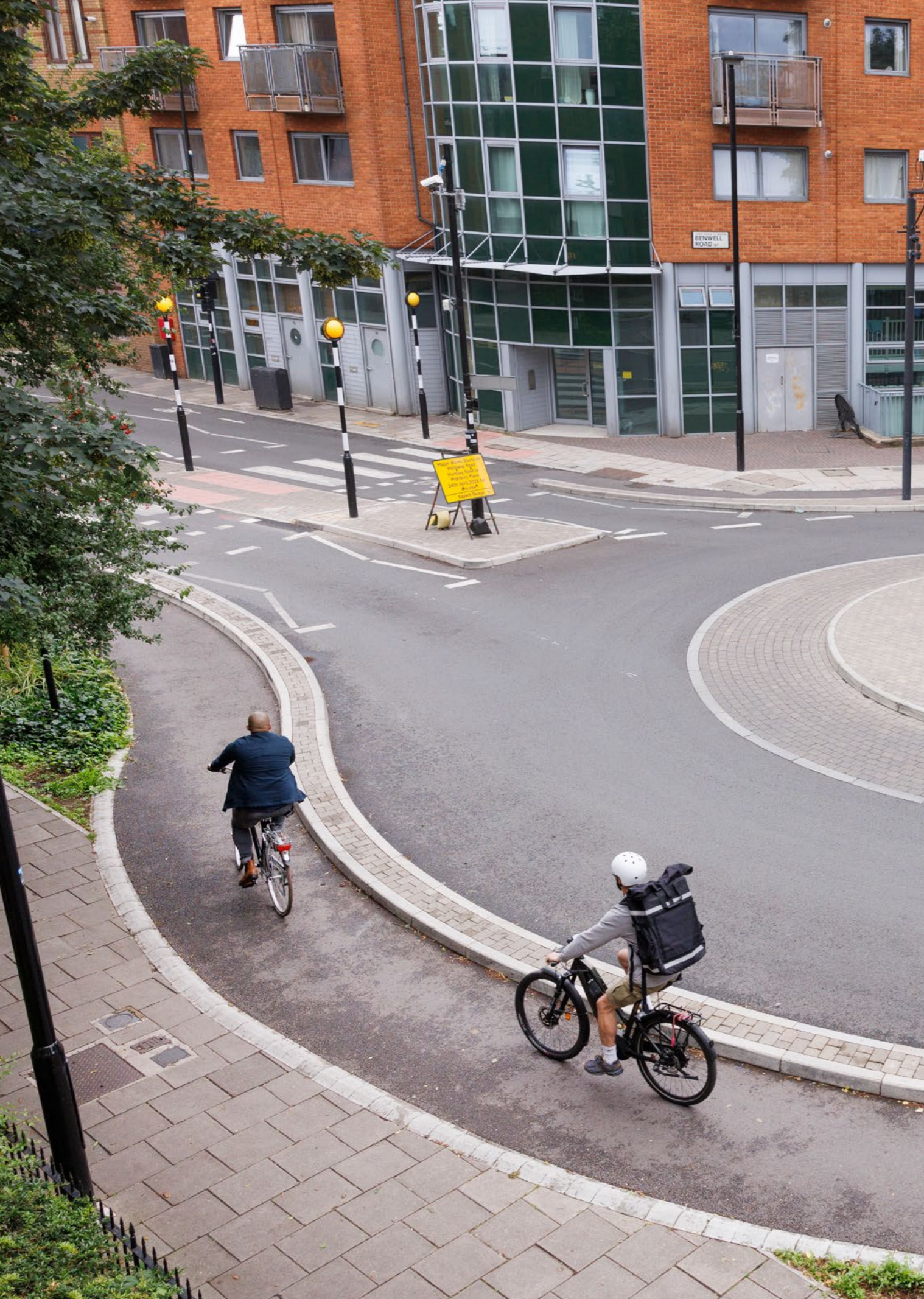
Segregated Cycleways are being constructed in several locations
